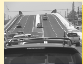
Traffic traverses the recently completed railroad overpass
